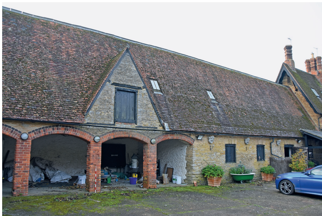
Figure 21: Turvey, Priory Farm- North elevation of the Stables and Cart Shed, looking south-west
