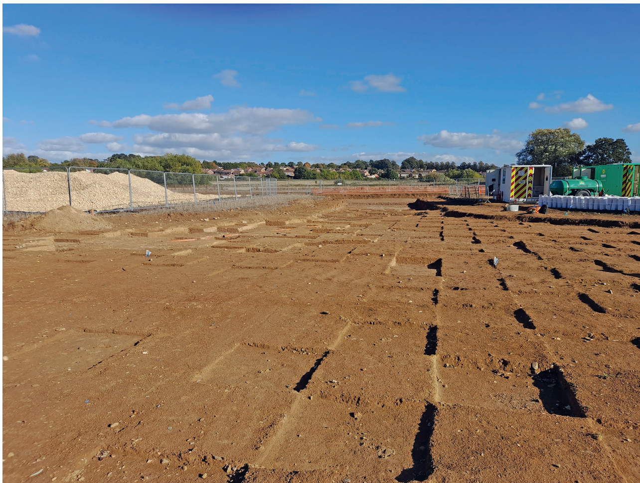
Figure 15: Flint-bearing layer on Northampton North West Relief Road, partly excavated (Oxford Archaeology)
