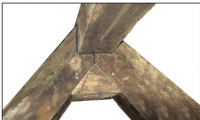
Figure 23: A fifteenth-century framed roof truss butt-apex joint with slip-tenon triangular block
